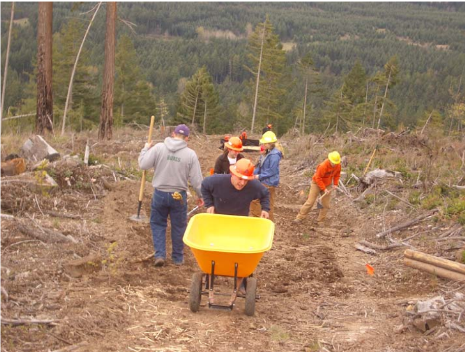
Students Prepare Site for Erosion Control Study
